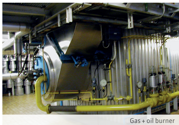
Gas turbine duct burner
