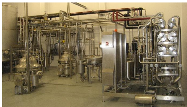
Technology for milk and whey treatment with reverse osmosis
